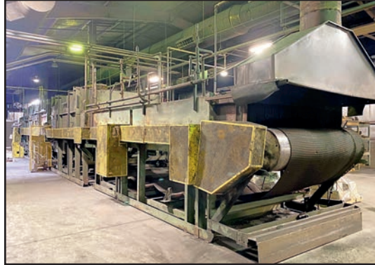
AFC-HOLCROFT NORMALIZING BELT TYPE ELECTRIC FURNACE SYSTEM
