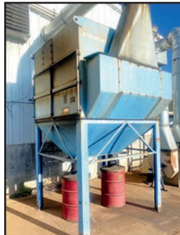
FARR TENKAY 20D DUST COLLECTOR
