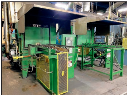
(2) DOW PRS304824 HEAT TREAT FURNACES
