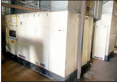
INGERSOLL RAND SSR-XFE300 300 HP ROTARY SCREW AIR COMPRESSOR
