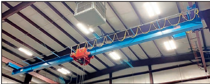
WAZEE 5-TON BRIDGE CRANE SYSTEM
