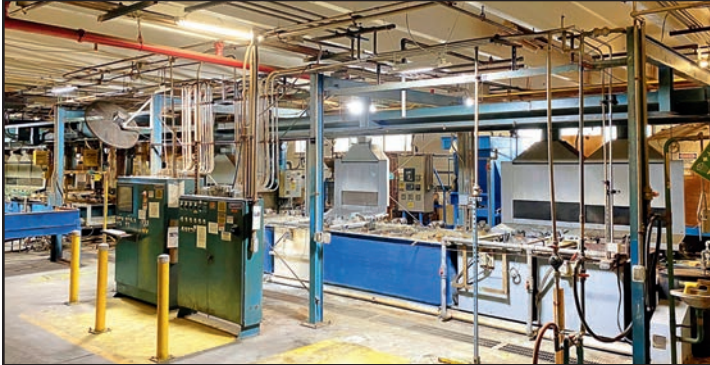
MABCO SYSTEMS NICKEL PLATING LINE
