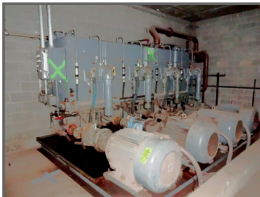
PUMP ROOM: (4) 100 HP WORLDWIDE ELECTRIC MOTORS; (4) PARKER DENISON P11V 2R5C 102A HYDRAULIC PUMPS AND TANKS
