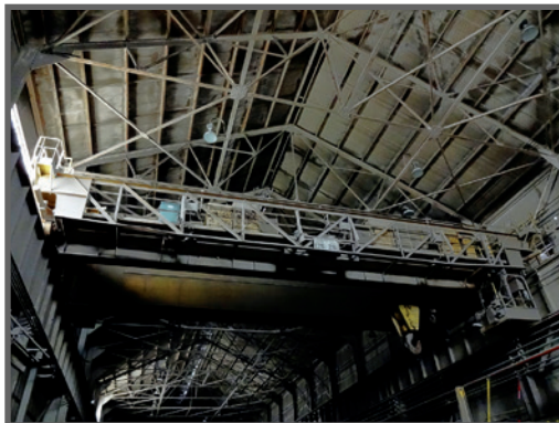
125 TON MORGAN BRIDGE CRANE
