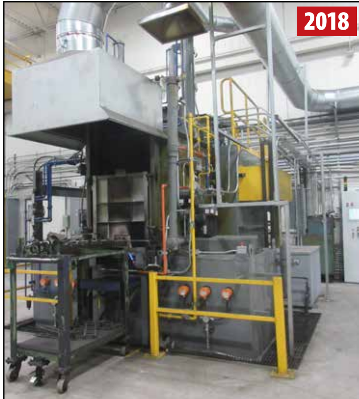
MIDLAND ROSS ALL-CASE 243624 LPG/METHANOL HEAT TREAT FURNACE
