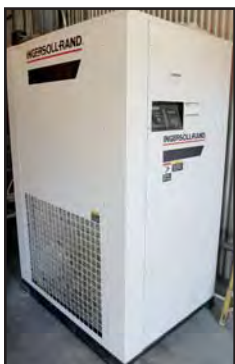
INGERSOLL RAND DXR800 REFRIGERATED AIR DRYER
