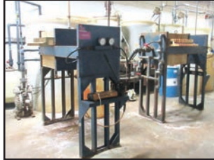
WASTE WATER TREATMENT PLANT
