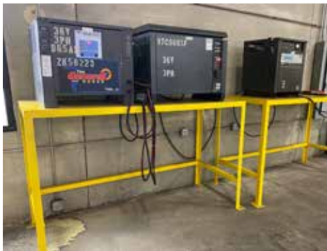
FORKLIFT BATTERY CHARGERS
