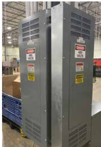
VIEW OF ELECTRICAL
