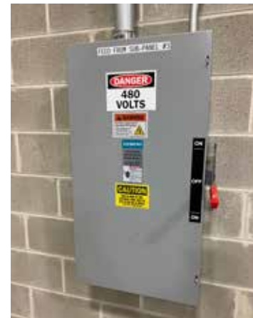
VIEW OF ELECTRICAL
