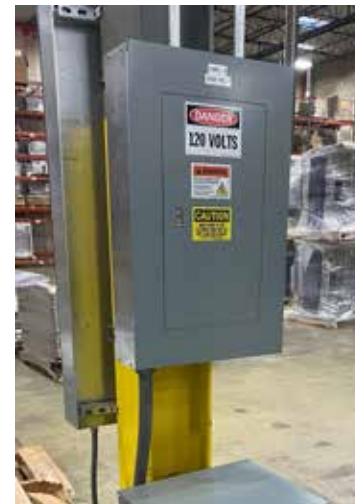
VIEW OF ELECTRICAL
