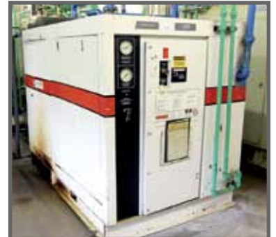
75 HP GARDNER DENVER ELECTRA-SAVER II COMPRESSOR
