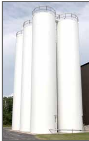
(6) PEABODY TECTANK 12' DIA. X 56' HIGH SILOS
