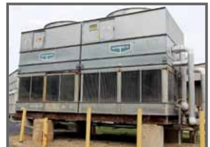
(2) EVAPCO ATW-278A WATER COOLERS
