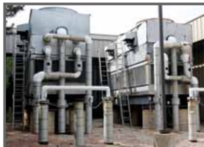
(2) EVAPCO ATW-135A WATER COOLERS
