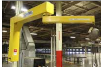
½ Ton GORBEL Jib Crane with Yale ½ Ton Hoist
