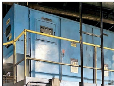
ESC INDUCTION IGBT800-1-3 800 KW INDUCTION HEATING SYSTEM
