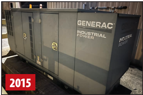
GENERAC 50 KW NATURAL GAS GENERATOR
