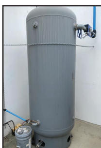
AIR RECEIVER TANK
