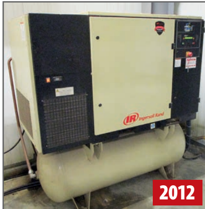
INGERSOLL RAND 30 HP AIR COMPRESSOR SYSTEM
