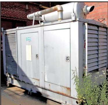
ONAN 230 0 DFP-17R-20074L ELECTRIC STAND-BY GENERATOR
