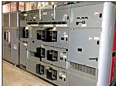
SQUARE D HLV-LOAD INTERRUPTER SWITCH UNIT AND POWER ZONE SWITCHGEAR
