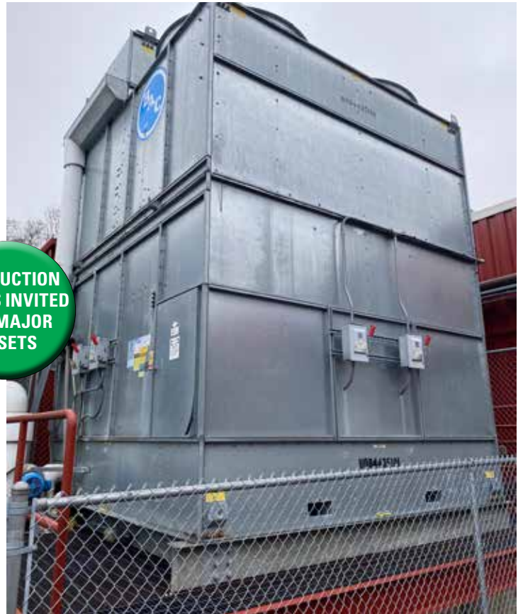
BAC FXV-643-20M COOLING TOWER
