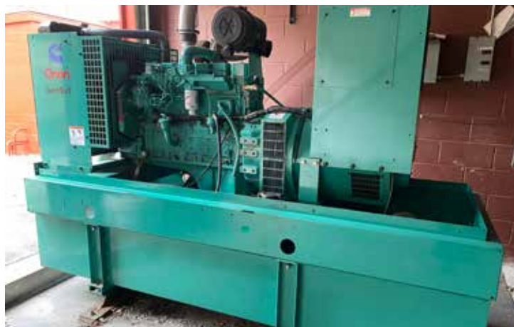
CUMMINS 80DGDA GENERATOR
