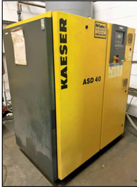
1 OF 2 KAESER ASD 40 ROTARY SCREW AIR COMPRESSORS
