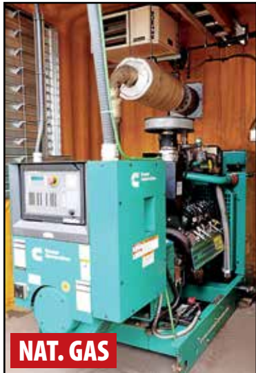
CUMMINS 100 KW GENERATOR
