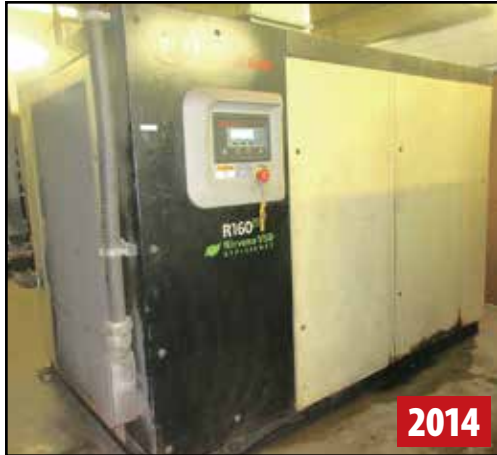
INGERSOLL RAND 200 HP AIR COMPRESSOR
