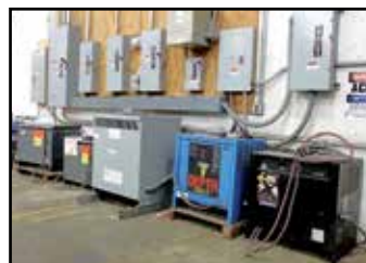
VIEW OF BATTERY CHARGERS
