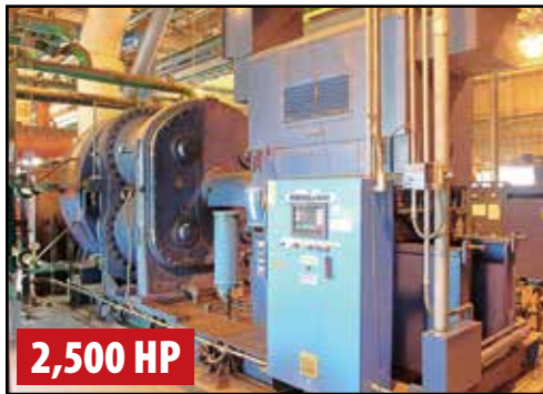
2,500 HP INGERSOLL RAND CENTAC CENTRIFUGAL AIR COMPRESSOR
