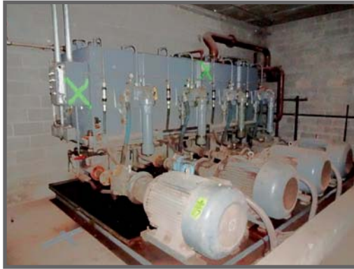
PUMP ROOM: (4) 100 HP WORLDWIDE ELECTRIC MOTORS; (4) PARKER DENISON P11V 2R5C 102A HYDRAULIC PUMPS AND TANKS
