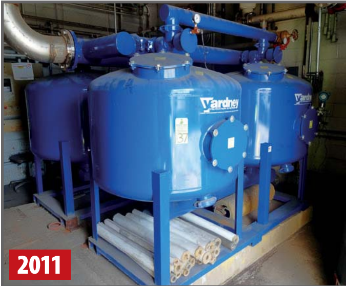
2011 YARDNEY RCW4824-4AS COOLING TOWER SAND MEDIA FILTER
