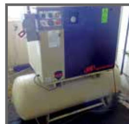
INGERSOLL RAND UP6-15C-125 ROTARY SCREW TYPE AIR COMPRESSOR
