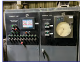
(above/left) East Side, 2500 Deg. F Custom Built Car Bottom Furnace, 216" W x 180" H x 300" D, natural gas fired, 10 burners, 2 zones, fiber lined, Honeywell controls with PLC
