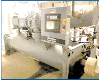
YORK MILLENNIUM SCREW CHILLER 200-TON PROCESS COOLING WATER CHILLER
