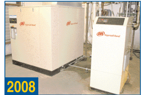
INGERSOLL RAND SSR-EP100 100-HP ROTARY SCREW AIR COMPRESSOR & INGERSOLL RAND NVC400A400 REFRIGERATED COMPRESSED AIR DRYER
